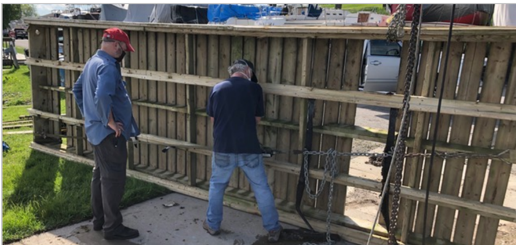
Mike Hope and Scott Creamer work to repair the main E-dock section that was damaged by ice during the winter. The section is now back in place and the dock as good as new.
