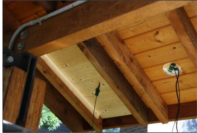
Figure B.33: Mailbox insulated
