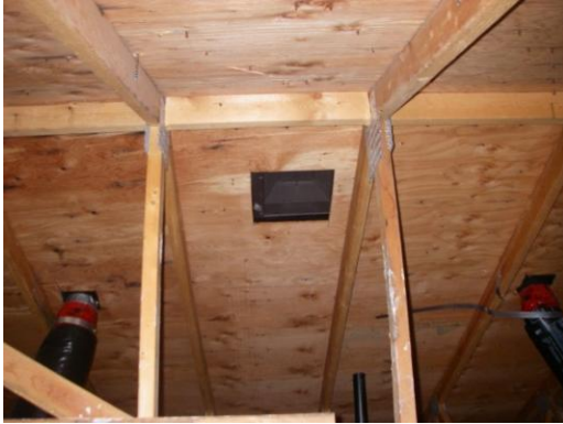
Photo 4: Roof Penetrations and Vent at Ridge
