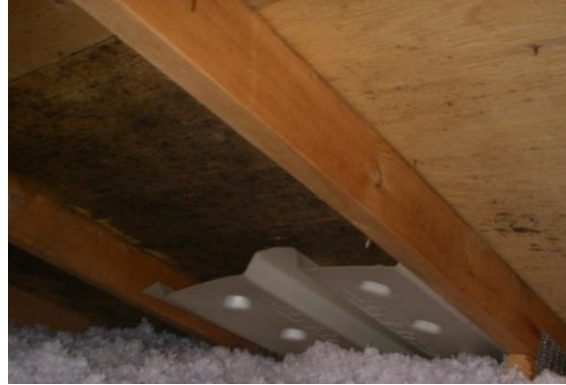
Photo 5: Baffle Vent at Soffit
