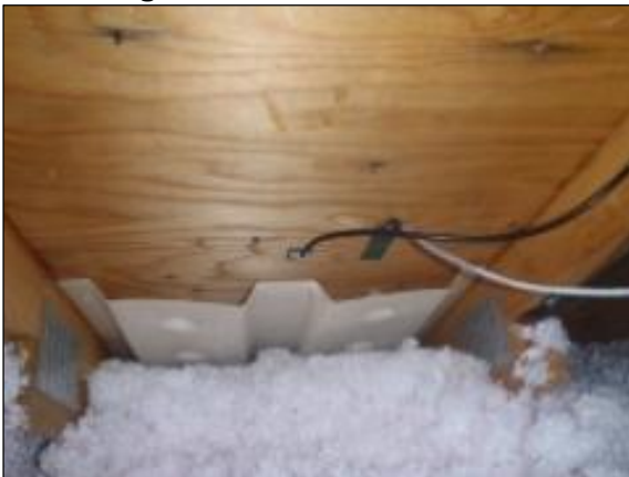
Figure B.11: Unit 2 west baffle
