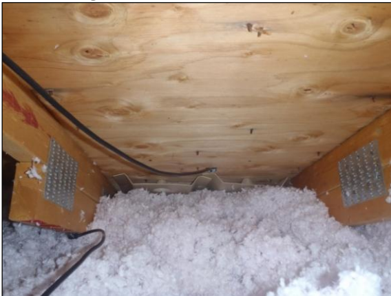
Figure B.3: Unit 1 west baffle
