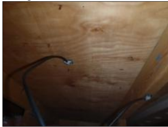
Figure B.28: Unit 4 west non-baffle
