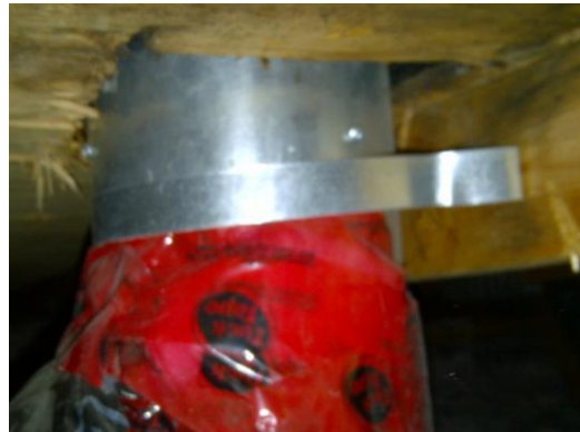
Photo 7: Air Barrier Sealing of Dryer Duct Penetration at Roof Sheathing
