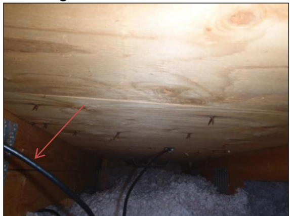
Figure B.21: Unit 3 east truss
