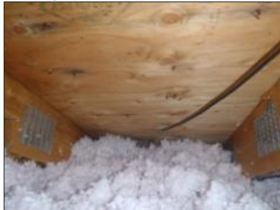
Figure B.4: Unit 1 west non-baffle
