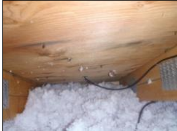
Figure B.2: Unit 1 east non-baffle
