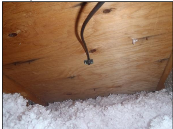
Figure B.20: Unit 3 west non-baffle
