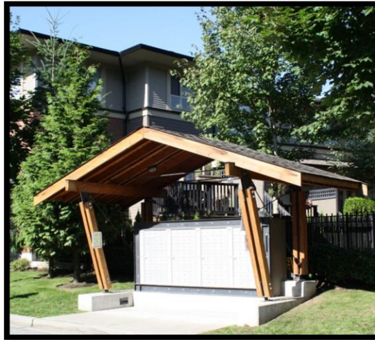
Photo 1: Test (Control) Roof Assembly with Unit 2 in the background
