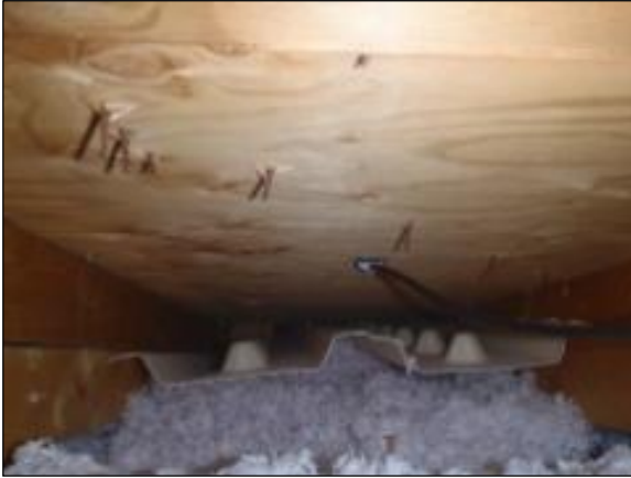
Figure B.17: Unit 3 east baffle
