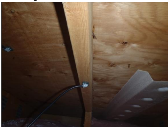
Figure B.29: Unit 4 south truss
