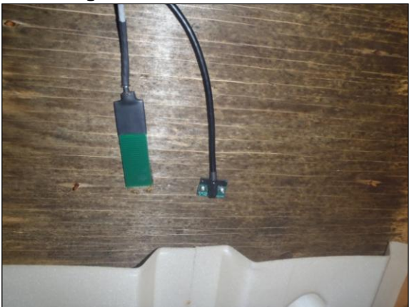
Figure B.19: Unit 3 west baffle
