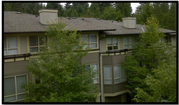
Photo 3: East Elevation of Unit 1
