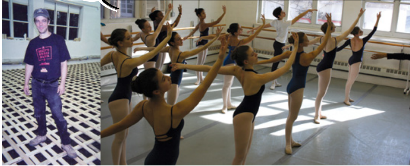
Technical Director Ted Bannigan overseeing construction of triple-sprung floors, only kind in borough. Designed at Texas A&M University School of Engineering, the system creates a dance floor with no direct x-y axis of impact, enabling impact of feet to be spread safely across staggered planes of x, y and z. Resistance and hard landings caused by a direct x-y axis are totally absent, to allow soft and bouncy landings. Try it. Where else can you dance in a backdrop of woodlands?
