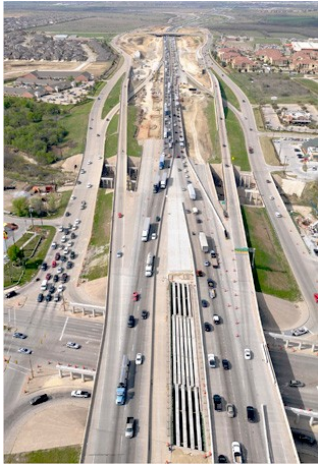
IH 35W Segment 3B – Under construction
