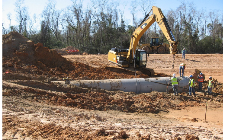
Closed Trunkline Drainage System
