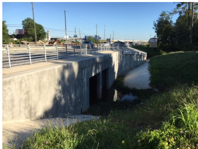
Multiple Box Culvert
