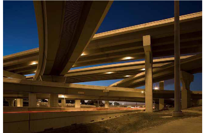
IH 10/IH 610 Interchange
