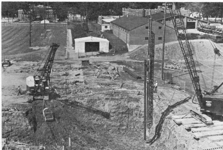
1. The ground is broken as the first piling is pounded in. And so the new addition begins.
